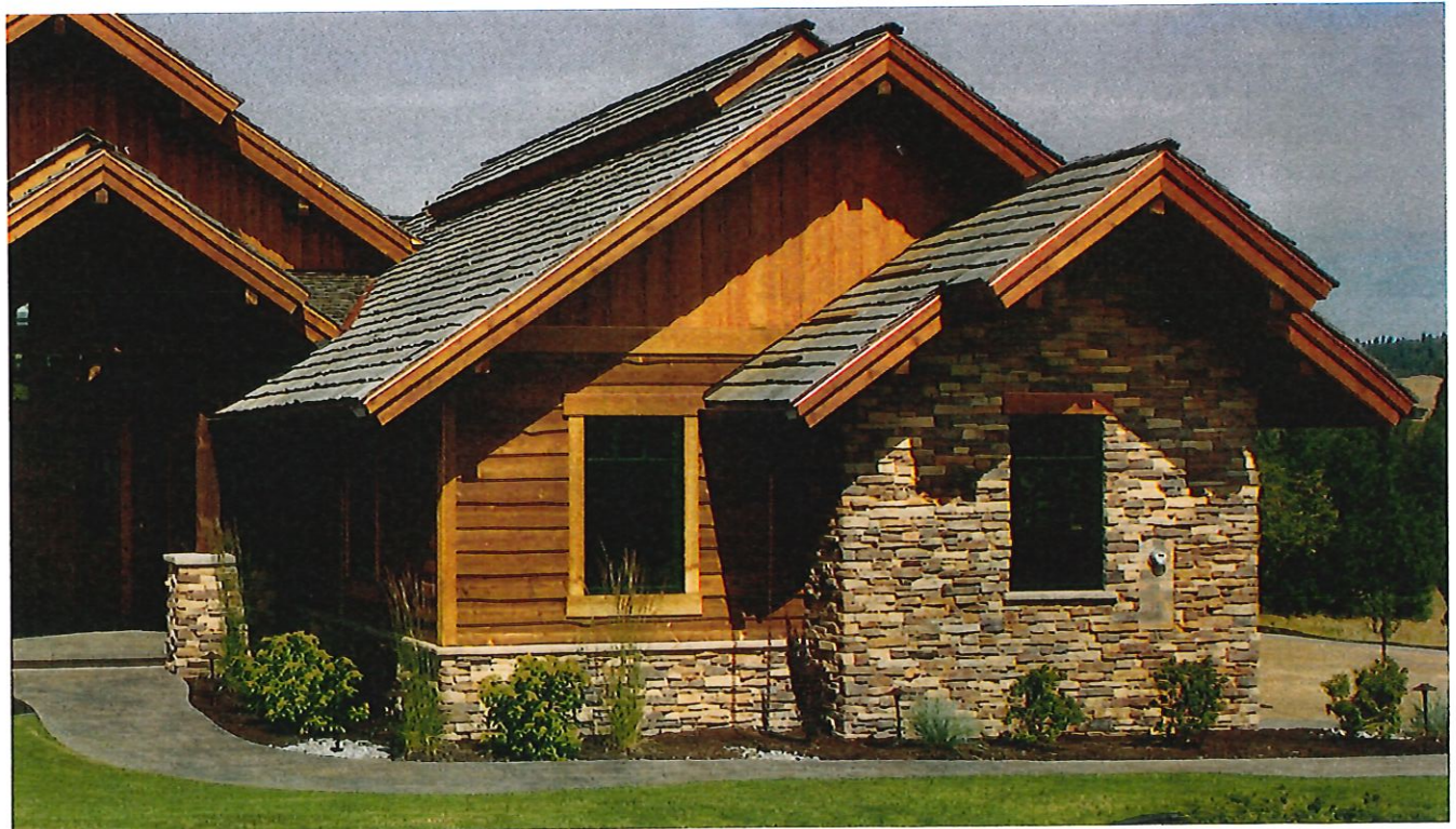
Durango Mountain Ledge using a dry-stack grout technique.
