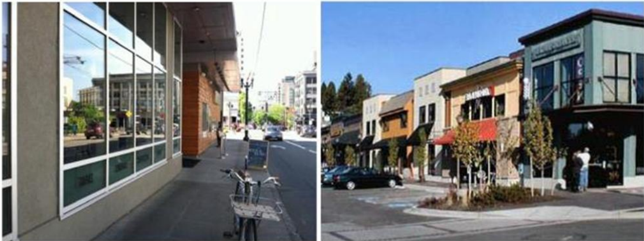
Figure 11: Examples of Change of Building Materials or Siding Style
