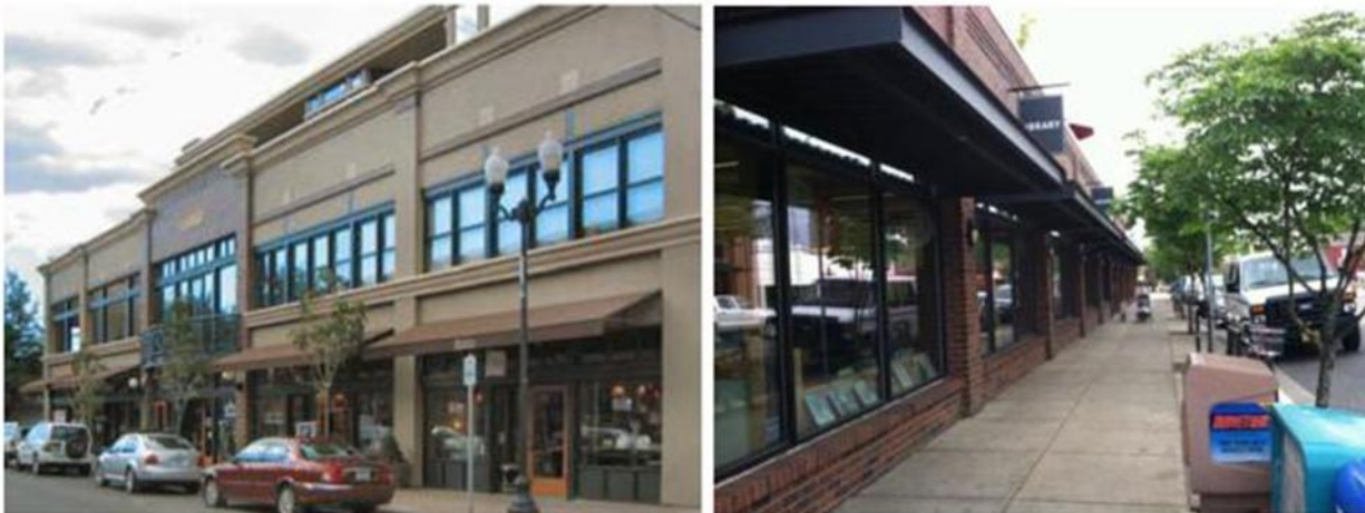
Figure 9: Examples of Buildings Using Distinct Window Patterns Separated by Other Elements, Such as Building Columns or Vertical Piers
